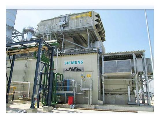
This Power Plant is composed of (3) of Gas Turbines (Siemens SGT-800) and (1) Steam Turbine (Siemens SST-900), (3) HRSG (Aalborg- Denmark), (1) ACC (SPX-Belgium), (1) RMS station, HV switchyard and BOP equipment including transformers, spare parts, control system, water conditioning system, etc.
